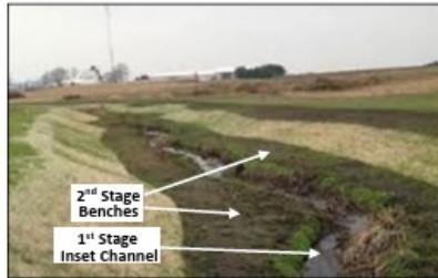
Figure 2. Constructed Two-Stage Ditch
